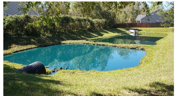
Retention Pond on the corner of Conner Grant and Adell. Photo Credit: Victoria Ferguson
